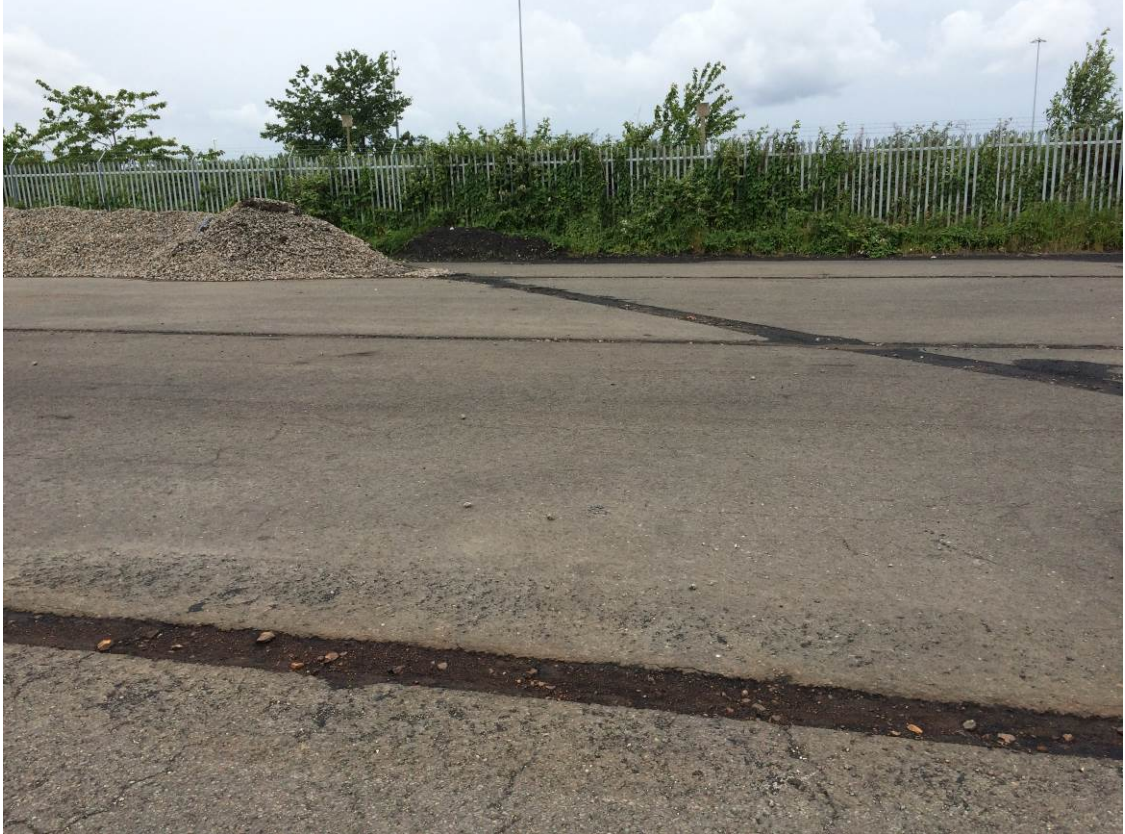
Photograph 2 – Hardstanding, rubble mound and fence line
